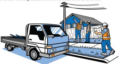
When operating machinery such as a digger or crane near lines you must keep at least four metres clear of overhead power lines.
