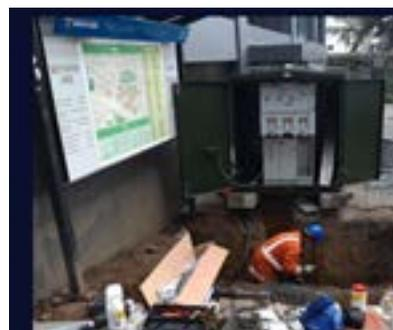
Mobile transformers have been successfully trialled as an alternative to diesel generation
