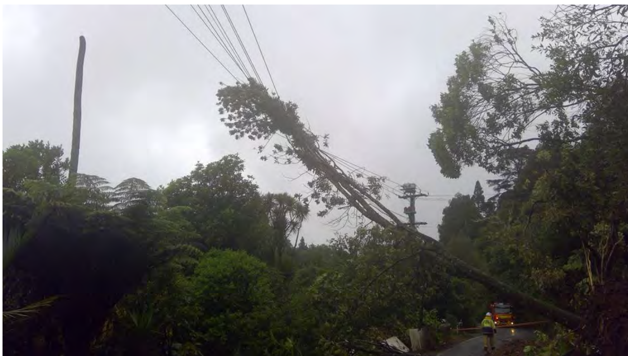
FIGURE 11.3: FALLEN TREE ON 11 KV OVERHEAD LINE AT ORATIA - FEBRUARY 2023
