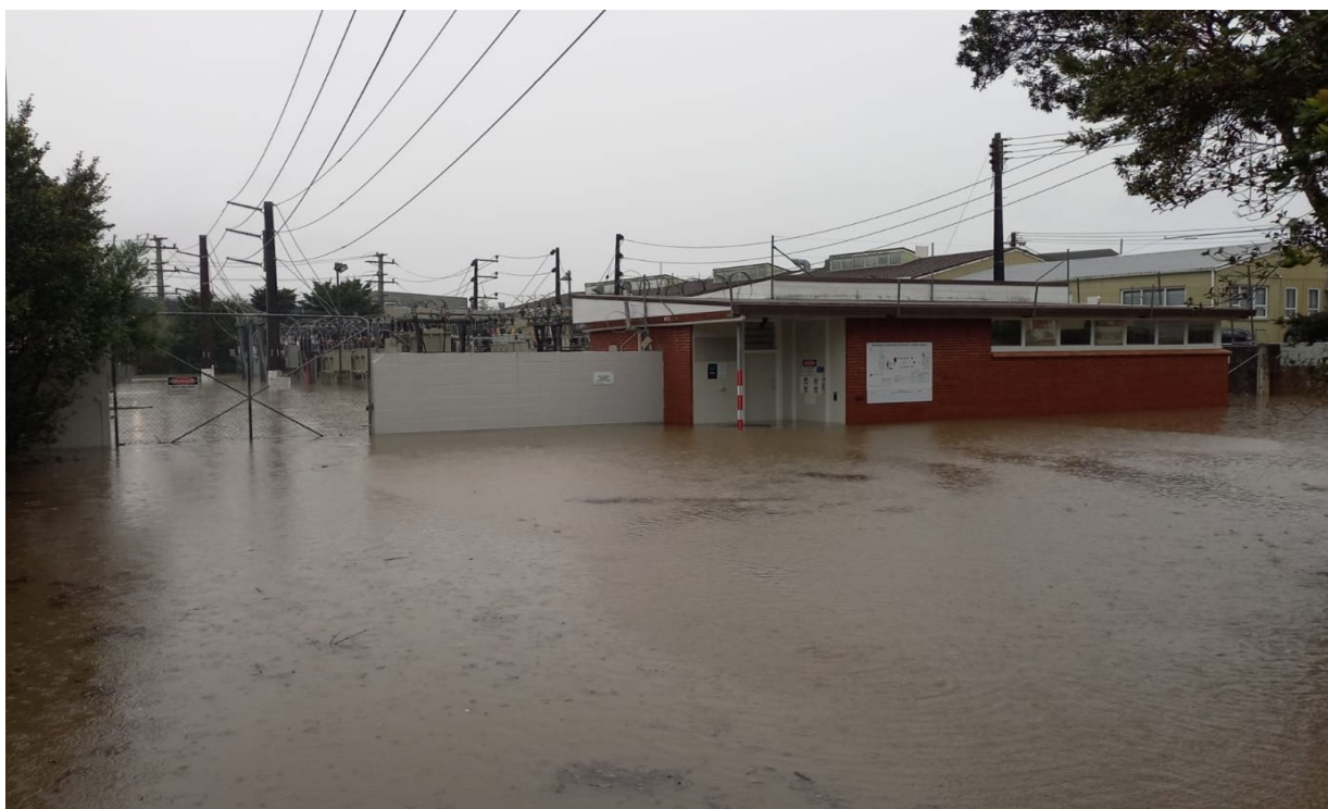
FIGURE 12A-1: WAIKAUKAU ZSS DURING FLOOD JANUARY 2023
