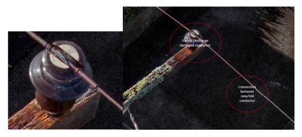
Reviewing the drone footage in conjunction with this acoustic information showed there was a partial discharge fault with this insulator causing aging to newly replaced conductor. It is the original insulator and was not replaced during a previous fault repair when the cable broke and fell. Originally the root cause was attributed to conductor but use of the new technology identified the actual cause and allowed for the correct remediation.
