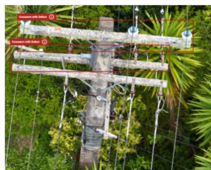
Pole conditions are annotated so an AI can learn how to do network inspections automatically
