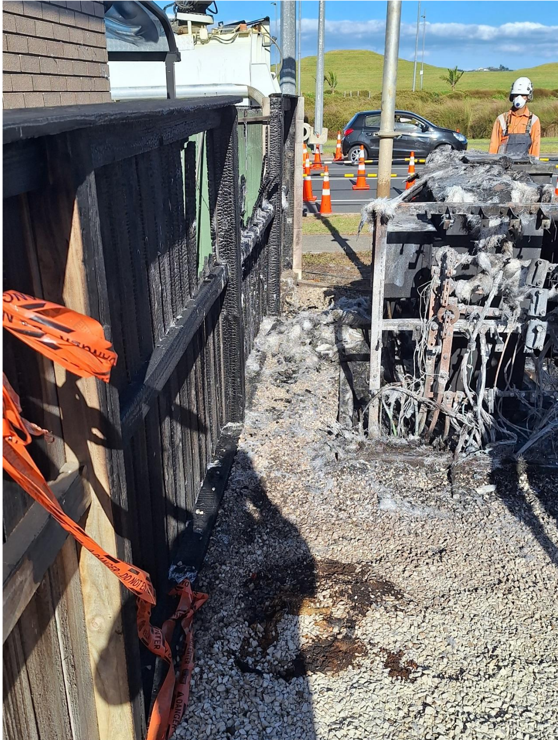
Figure 1: Transformer fire, Flatbush, Auckland
