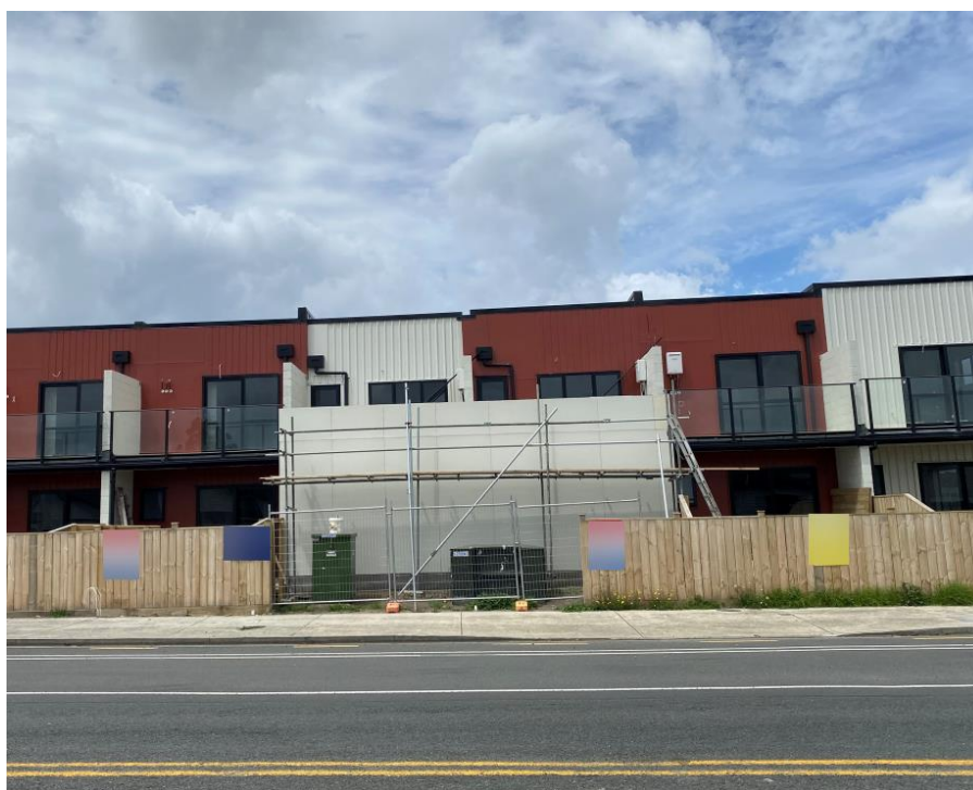
Figure 4: Non-compliant fire rated wall between new development and existing assets
