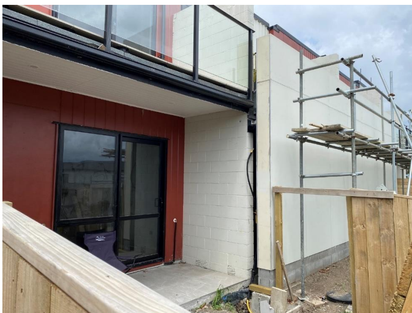
Figure 5: Units enclosed by fire wall
