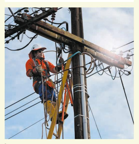
LINE MECHANIC WORKING ON DE-ENERGISED HIGH VOLTAGE LINES.
