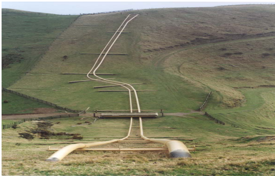
Figure 3-3 : Pipelines at Gibbs Fault near Wellington
