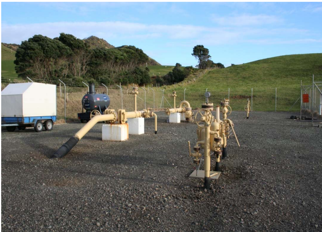
Figure 3-22 : Typical PIG launcher and receiver
