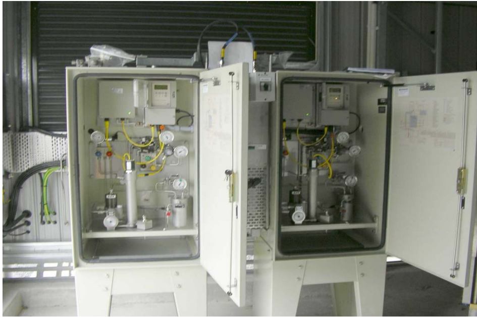
Figure 3-11 : Twin pumped odorant injection system
