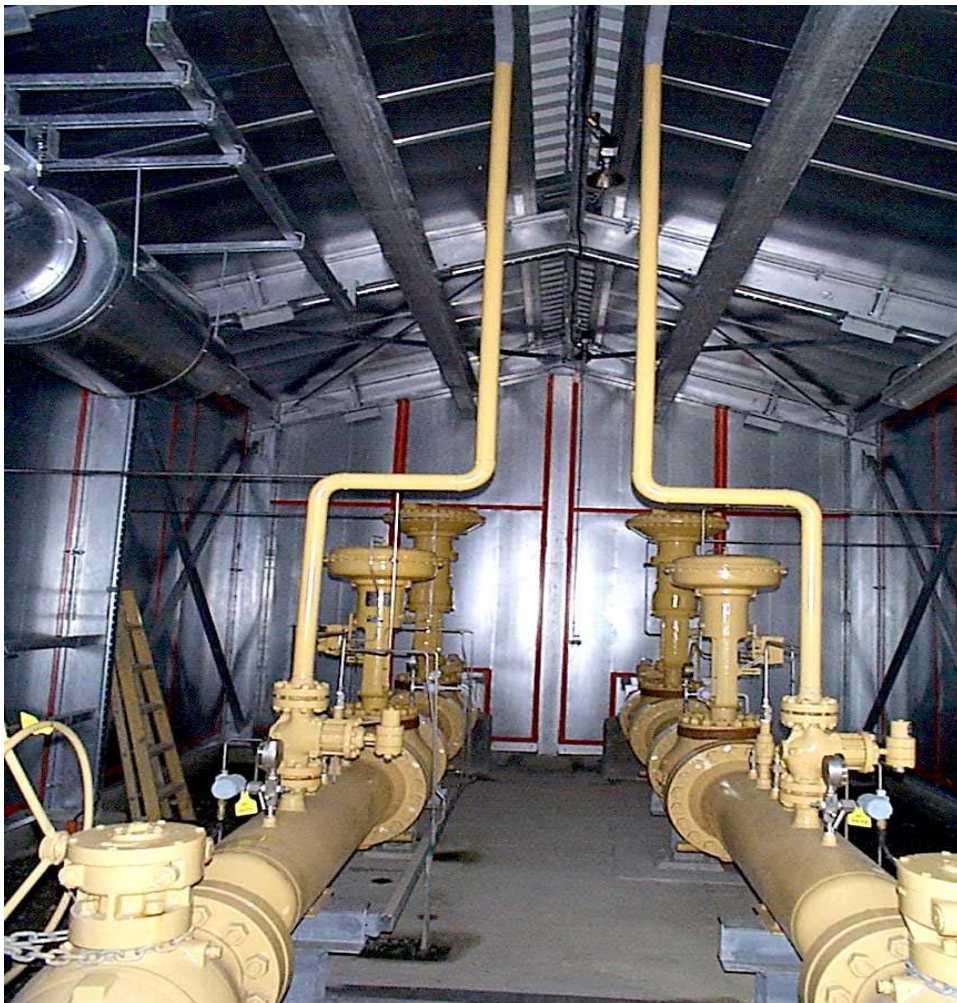
Figure 3-25 : Fisher pressure control valves
