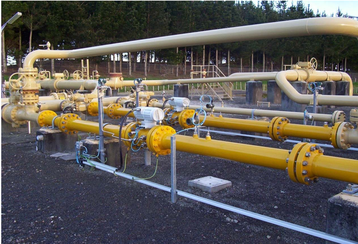
Figure 3-16 : Typical ultrasonic metering system
