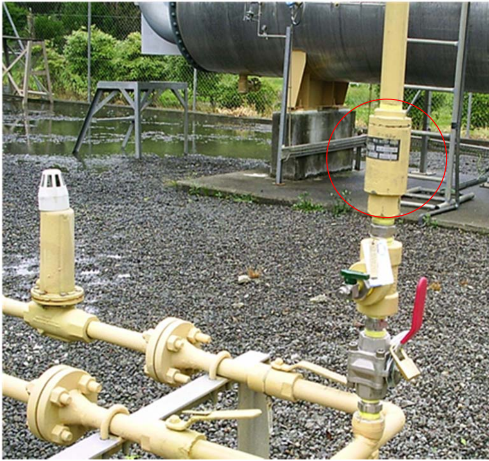
Figure 3-27 : Reliance pressure relief valve
