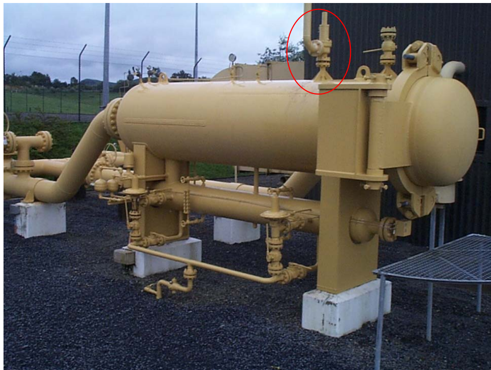
Figure 3-28 : Typical pressure relief valve fitted to a pressure vessel
