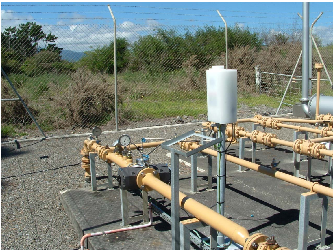
Figure 3-17 : Typical rotary displacement metering system
