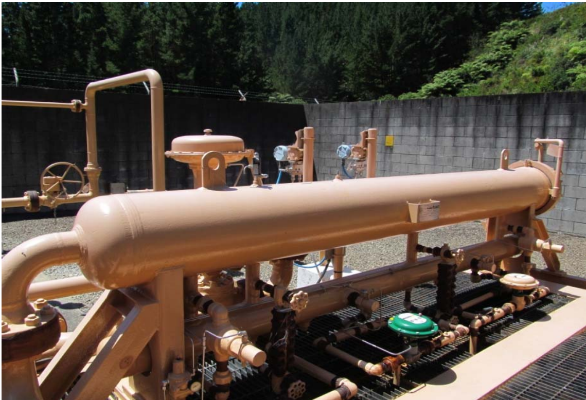
Figure 3-15 : Typical filter separator
