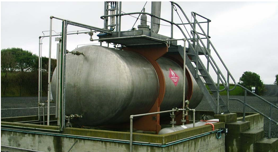
Figure 3-12 : Bulk odorant storage vessel
