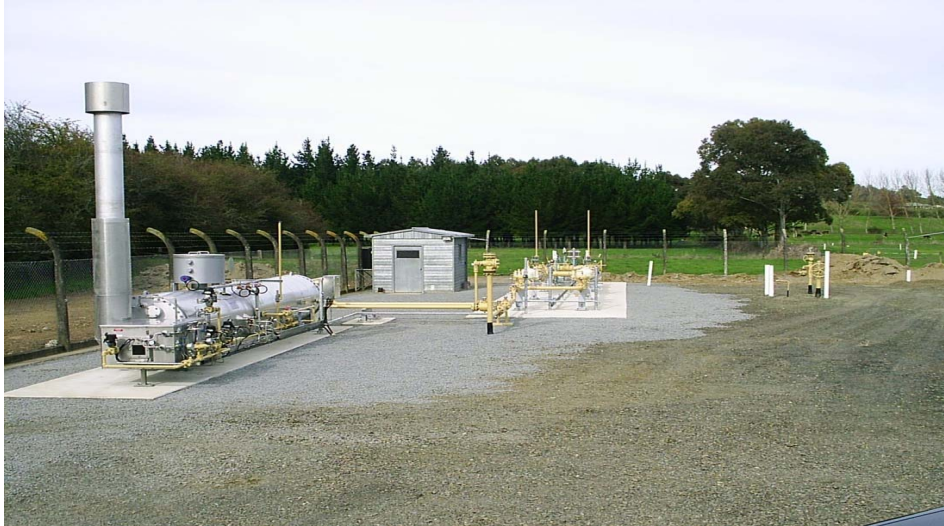
Figure 3-6 : Typical delivery point
