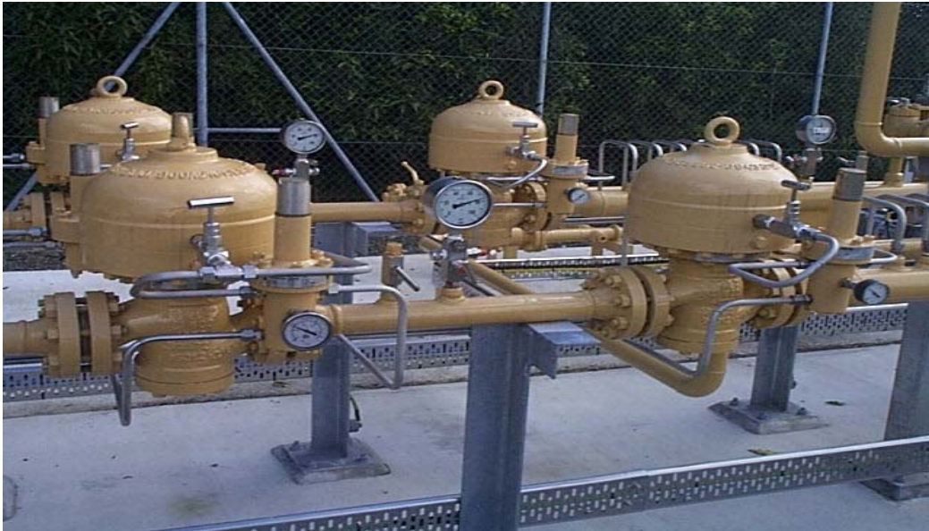
Figure 3-24 : Gortor pressure regulators
