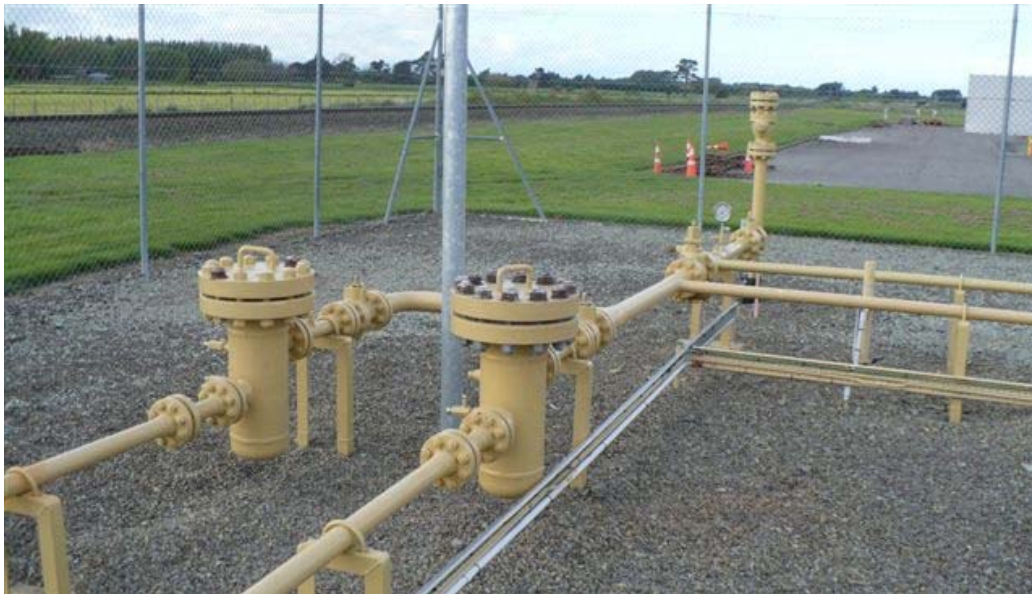
Figure 3-33 : Two typical filters
