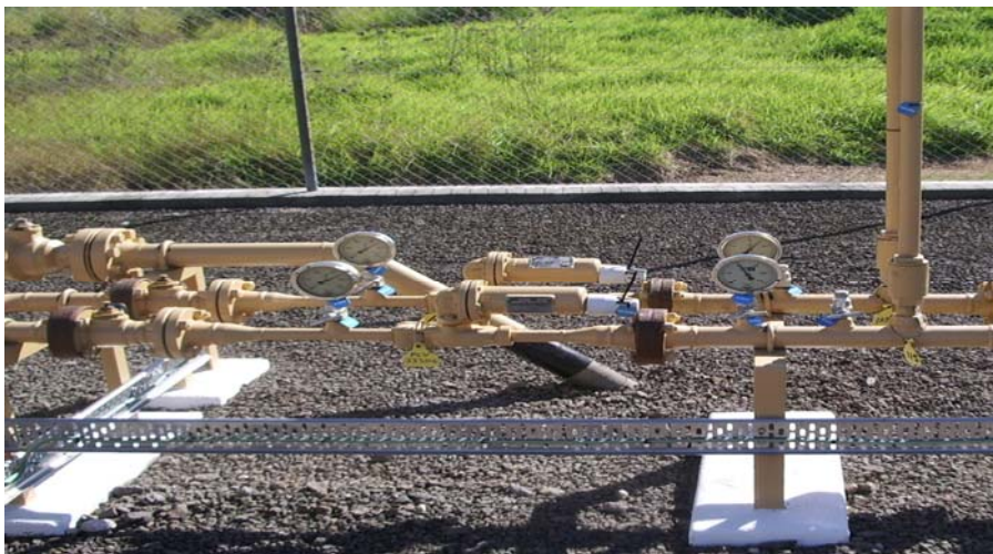
Figure 3-23 : Fisher 630 pressure regulators in typical twin stream configuration
