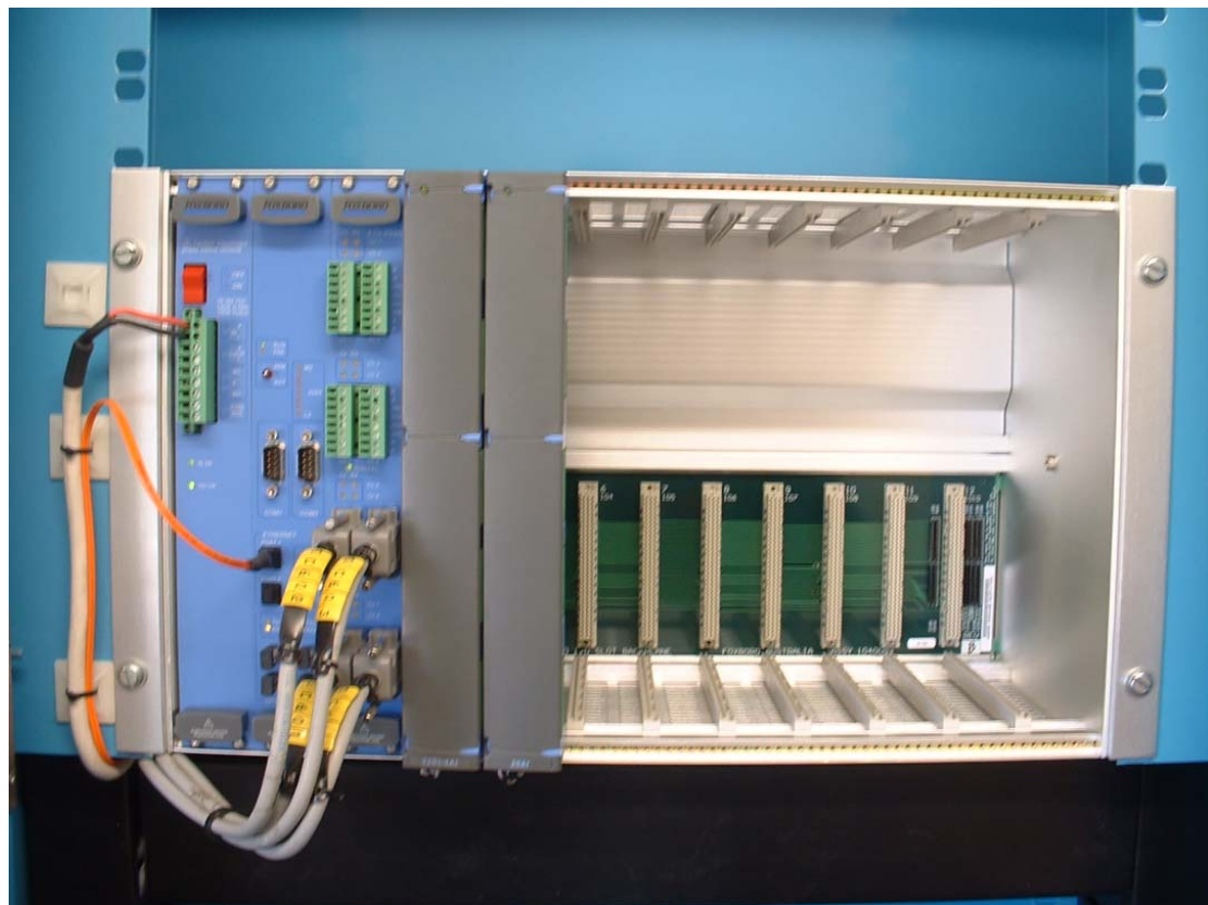
Figure 3-20 : Typical remote RTU cabinet
