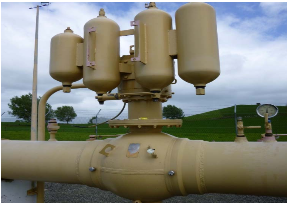
Figure 3-8 : Typical NB 400mm manually operated MLV
