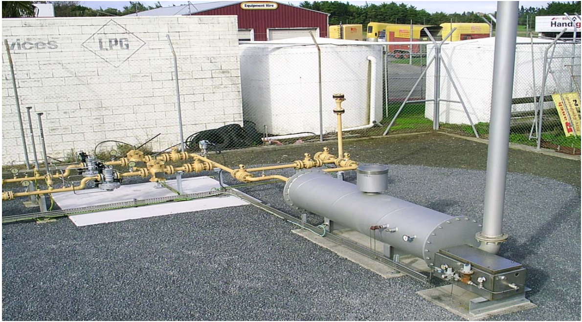
Figure 3-9 : Typical WBH installation
