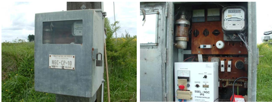
Figure 3-4 : Typical pole mounted rectifier unit
