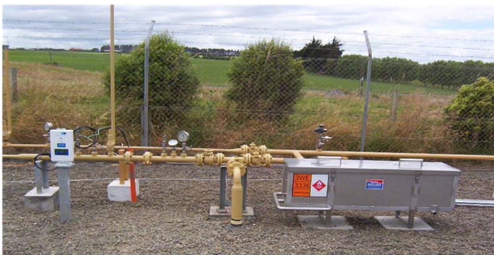
Figure 3-13 : Mobile bypass odorant unit
