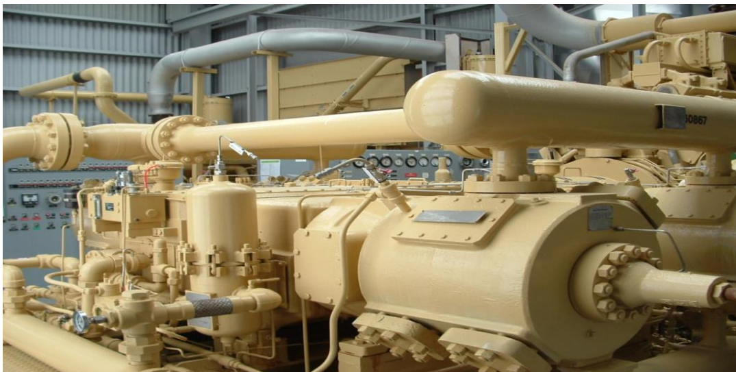
Figure 3-5 : Typical reciprocating gas compressor
