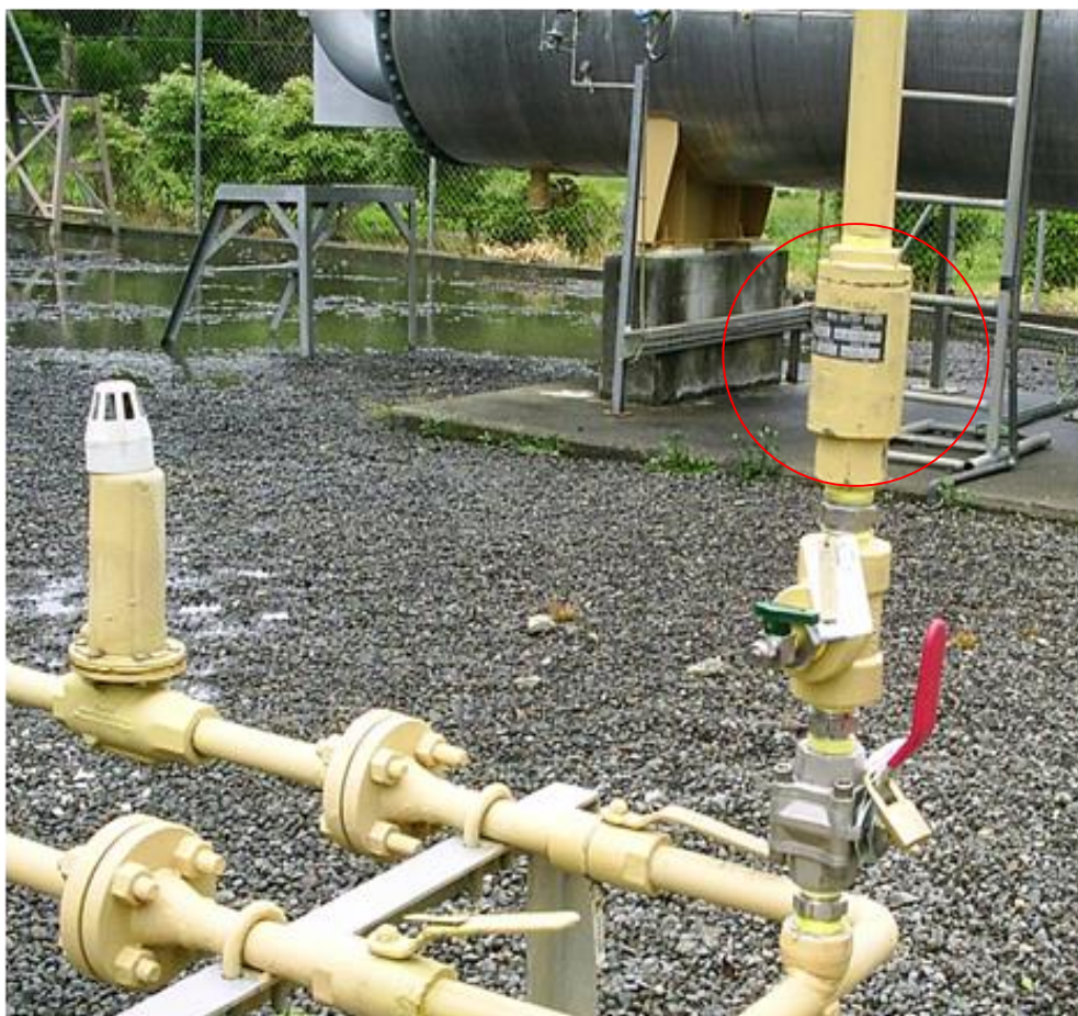
Figure 3-27 : Reliance pressure relief valve
