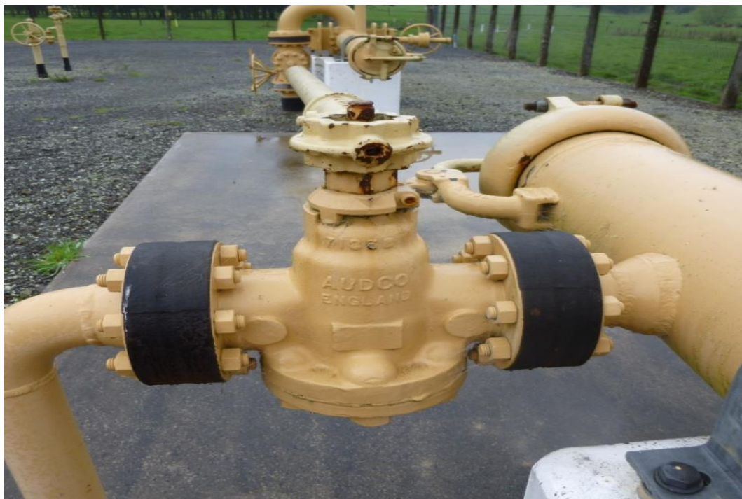
Figure 3-32 : A typical NB 50mm plug type isolation valve
