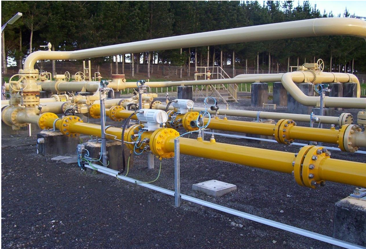
Figure 3-16 : Typical ultrasonic metering system
