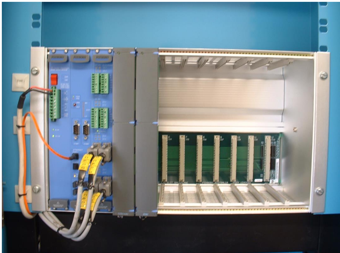
Figure 3-20 : Typical remote RTU cabinet
