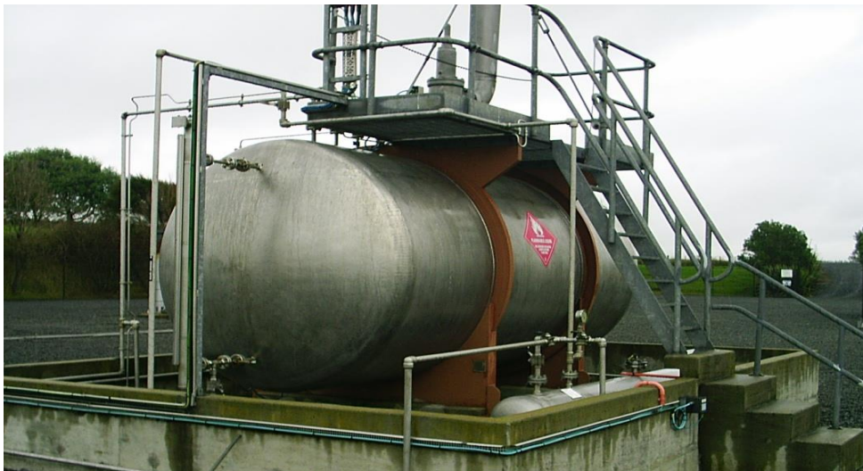
Figure 3-12 : Bulk odorant storage vessel
