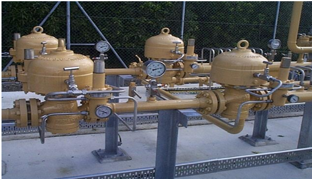
Figure 3-24 : Gorter pressure regulators
