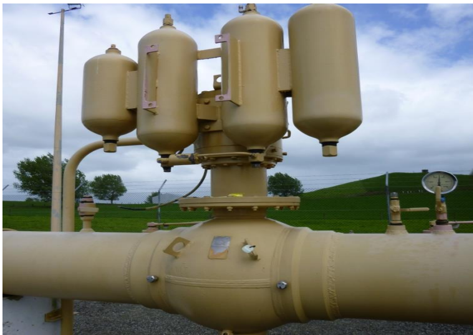
Figure 3-8 : Typical NB 400mm manually operated MLV
