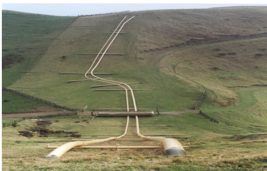
Figure 3-3 : Pipelines at Gibbs Fault near Wellington
