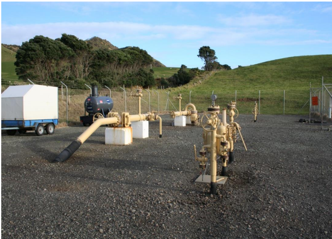
Figure 3-22 : Typical PIG launcher and receiver
