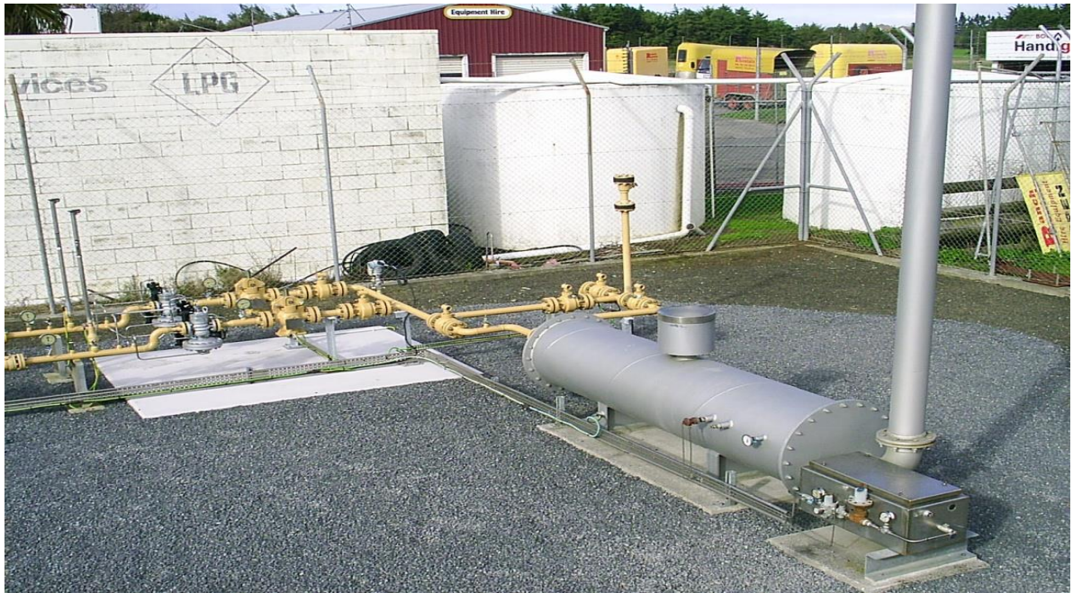
Figure 3-9 : Typical WBH installation
