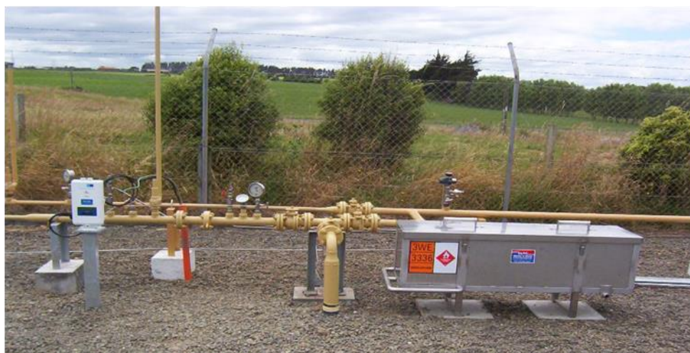
Figure 3-13 : Mobile bypass odorant unit
