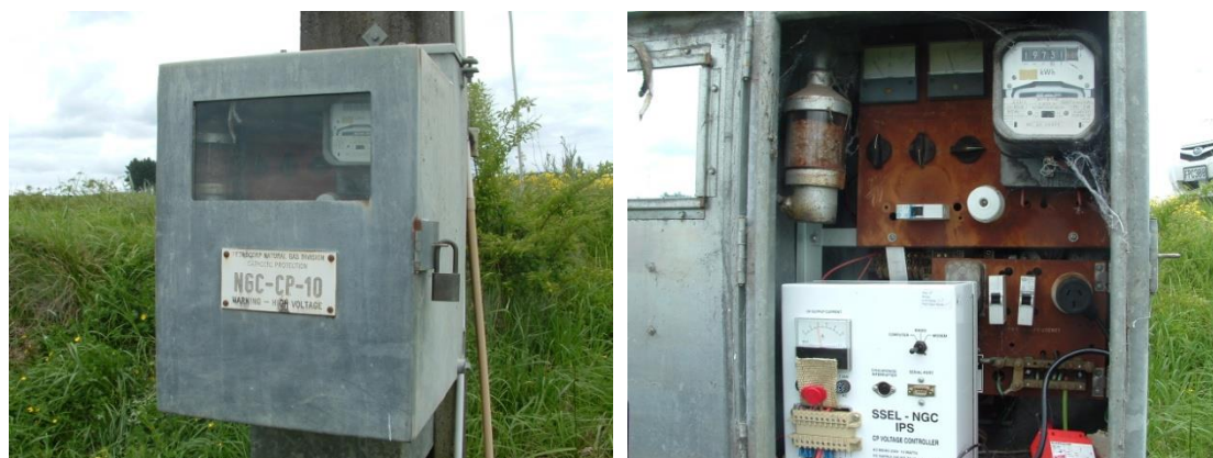
Figure 3-4 : Typical pole mounted rectifier unit
