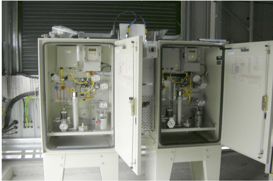
Figure 3-11 : Twin pumped odorant injection system
