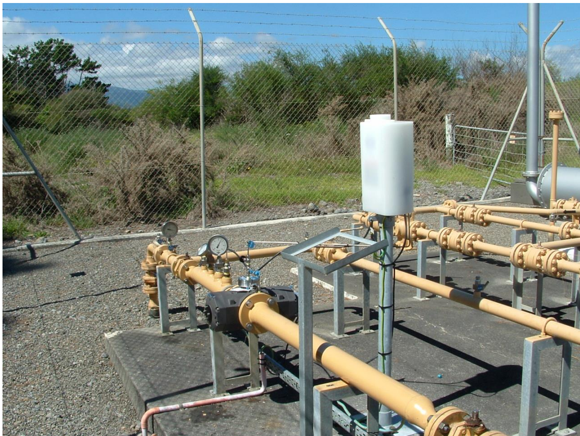
Figure 3-17 : Typical rotary displacement metering system
