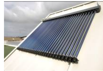
Hills evacuated tube solar hot water heater
