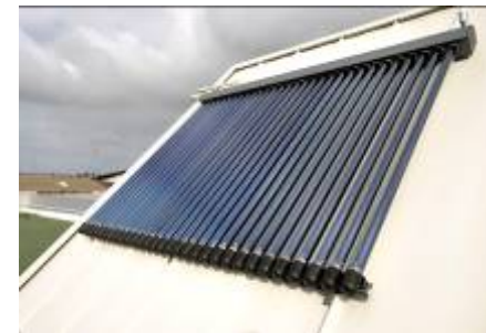
Hills evacuated tube solar hot water heater
