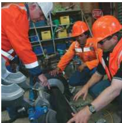
A Utilitech gas trainer delivers 'hands on' training on polyethylene pipe butt jointing at a client's premises.
