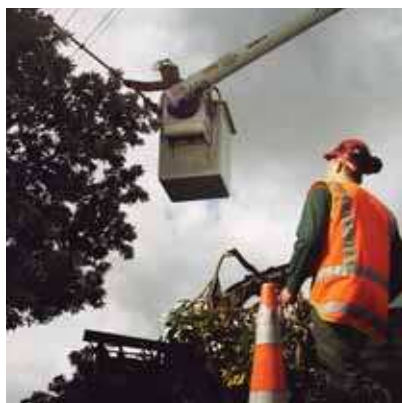
Keeping trees clear of lines is one of the methods Vector uses to maintain network reliability.
