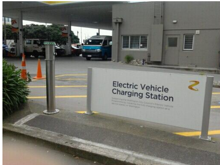
Figure 1. An electric vehicle charging station in Wellington
